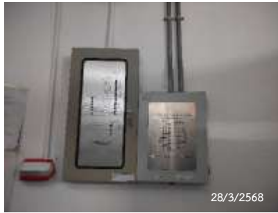
Graphic Annunciator Fire Alarm System
