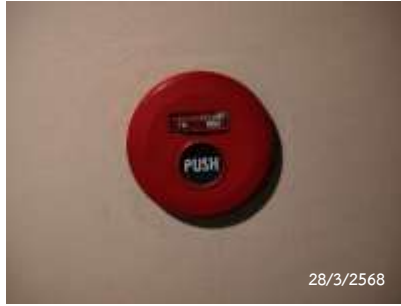
Fire Alarm Manual Station
